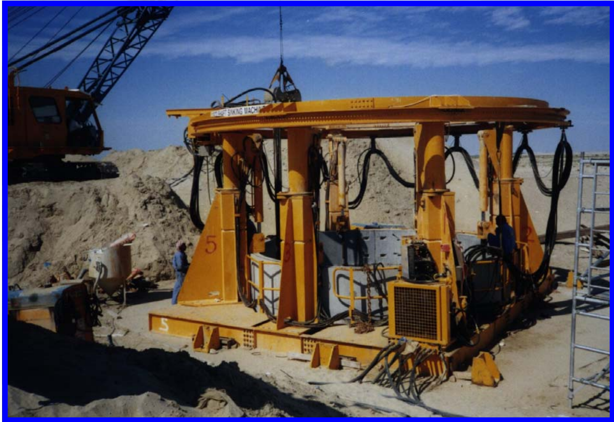
SHAFT SINKING MACHINE at work in DUBAI
